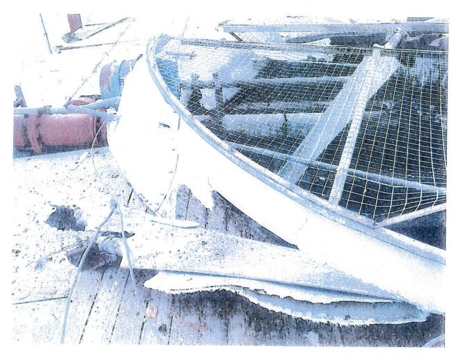
Fig. 8 – Damage to Cooling Tower #1
