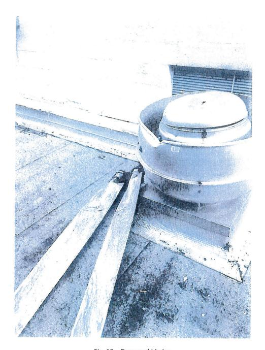
Fig. 10 – Damaged blades
