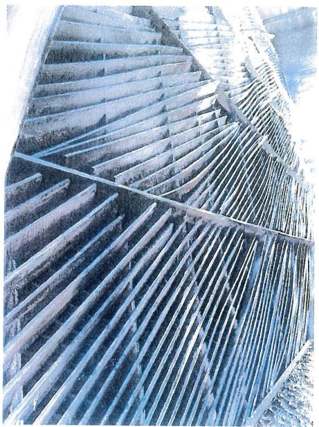
Fig. 5 – Inside view of Cooling Tower wooden fill
